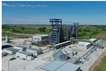
Monolith uses 100 percent renewable electricity to produce "green" carbon black and clean hydrogen, which can be converted to clean ammonia. Target applications include molded parts for auto interiors and underhood. The process reportedly reduces greenhouse gas emissions 90 percent. Courtesy of Monolith
